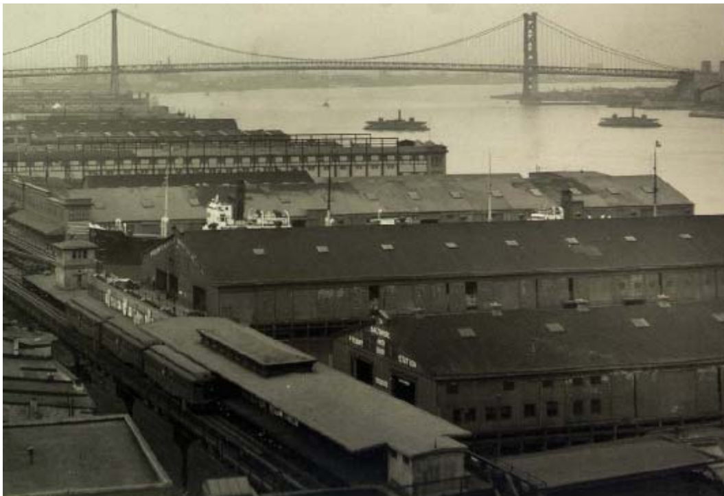
Delaware Avenue looking North toward Ben Franklin Bridge
