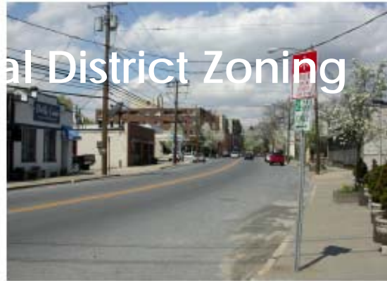
Fig. 5.1 Hope Street looking north, existing conditions
