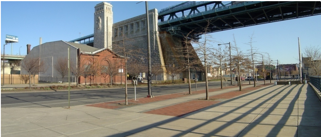
Columbus Boulevard and Water Department site
