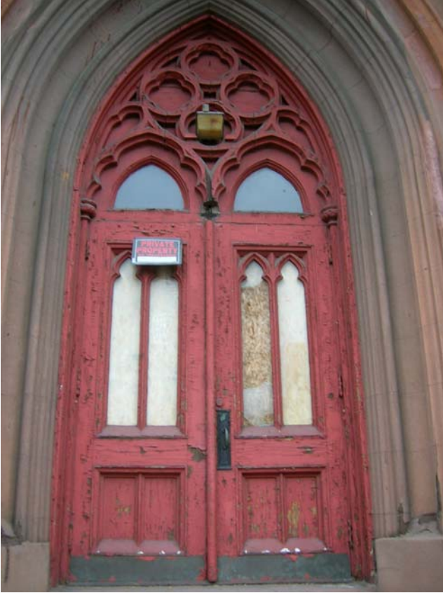
Figure 5. Church of the Assumption, south elevation entrance. March 2009. (Photographs by author)
