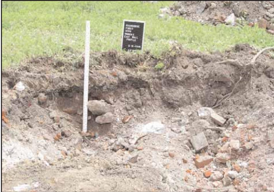
**Photograph 13:** Shot of east wall profile of Beach Street Power Station Trench 3 showing demolition fill and impenetrable steel reinforced concrete in Historic Area H-1. View facing east (May 2008).
