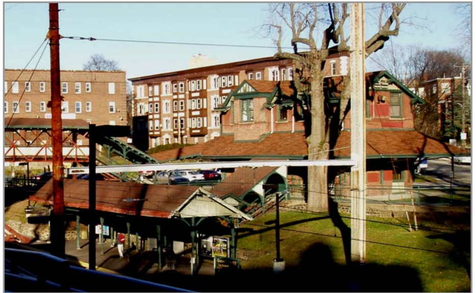
Queen Lane Train Station
