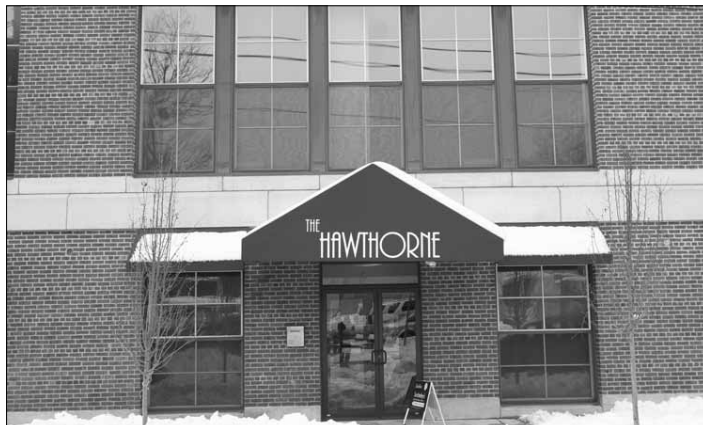
The old Hawthorne School, built in 1909, was recently converted to luxury loft-style apartments. Harvey Finkle
