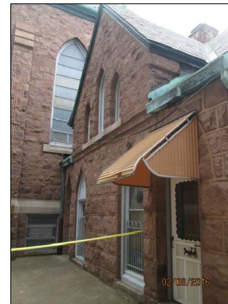
VIEW FROM COURTYARD LOOKING EAST
