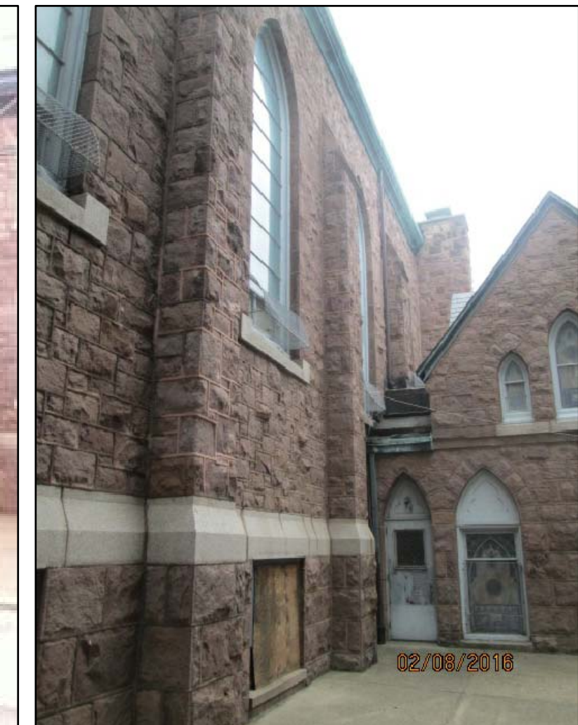
VIEW FROM COURTYARD LOOKING SOUTH
