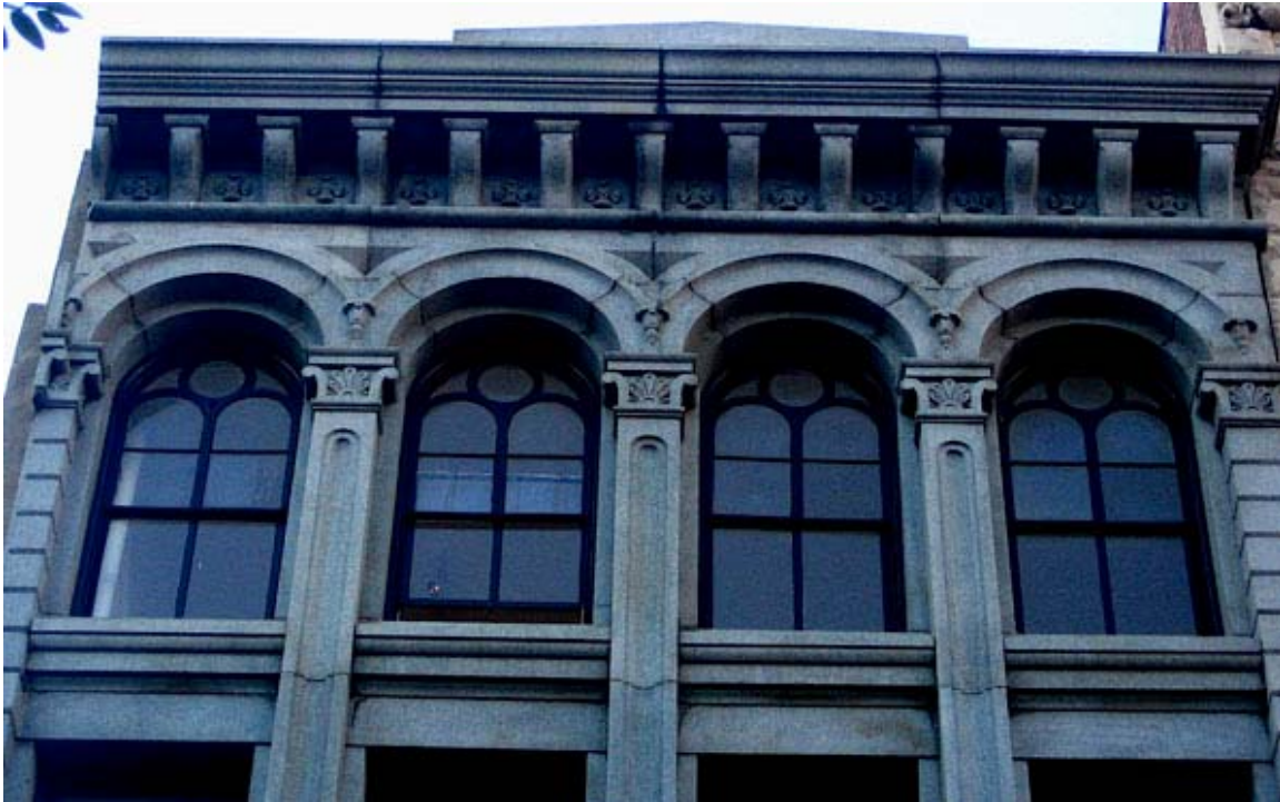
Figure 2 (above): Cornice and fourth floor detail of Chestnut Street elevation.
