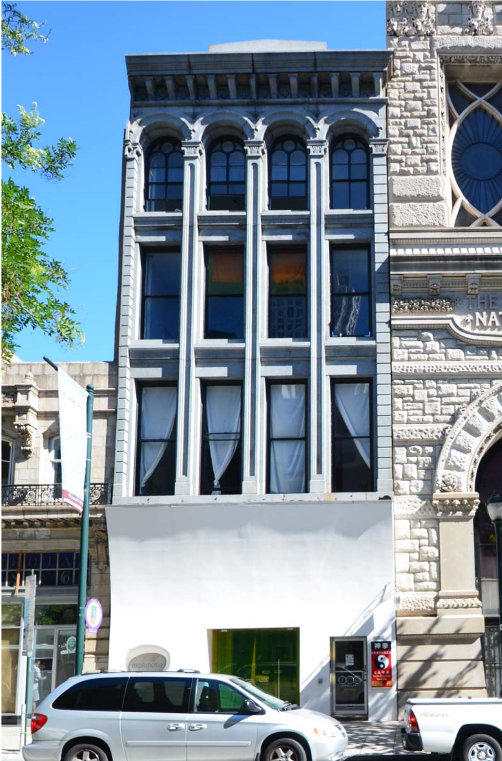
Figure 1: South (Chestnut Street) elevation.
