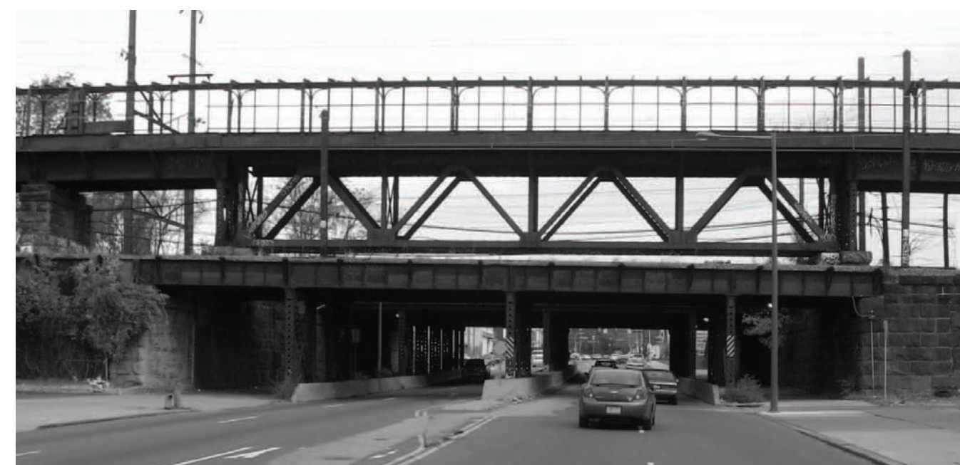
Existing: 52nd Street rail underpass
