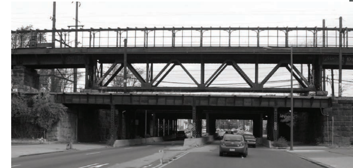
E. Existing: 52nd Street rail underpass
