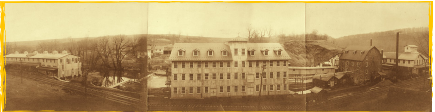
A panoramic view of the mill looking east, taken from across the railroad tracks in 1961. Do you see the back of the old stone mill on the right and the dam and head race on the left?
